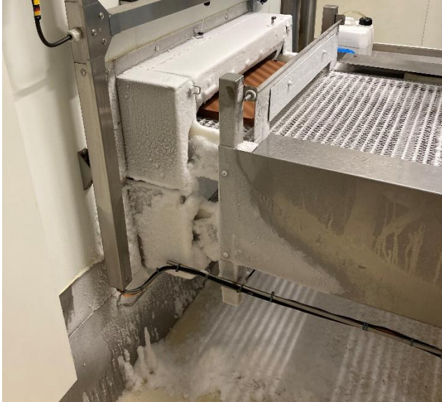
Figure 9: accumulation excessive de givre
